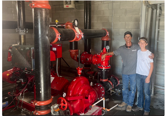
Gray-Salmon's husband, Ray, and oldest son, Bodie, on the job at Foothill Fire.
